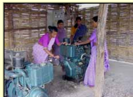
Electricity generation using Pongamia oil at Chalpadi hamlet, Adilabad District, Andhra Pradesh
